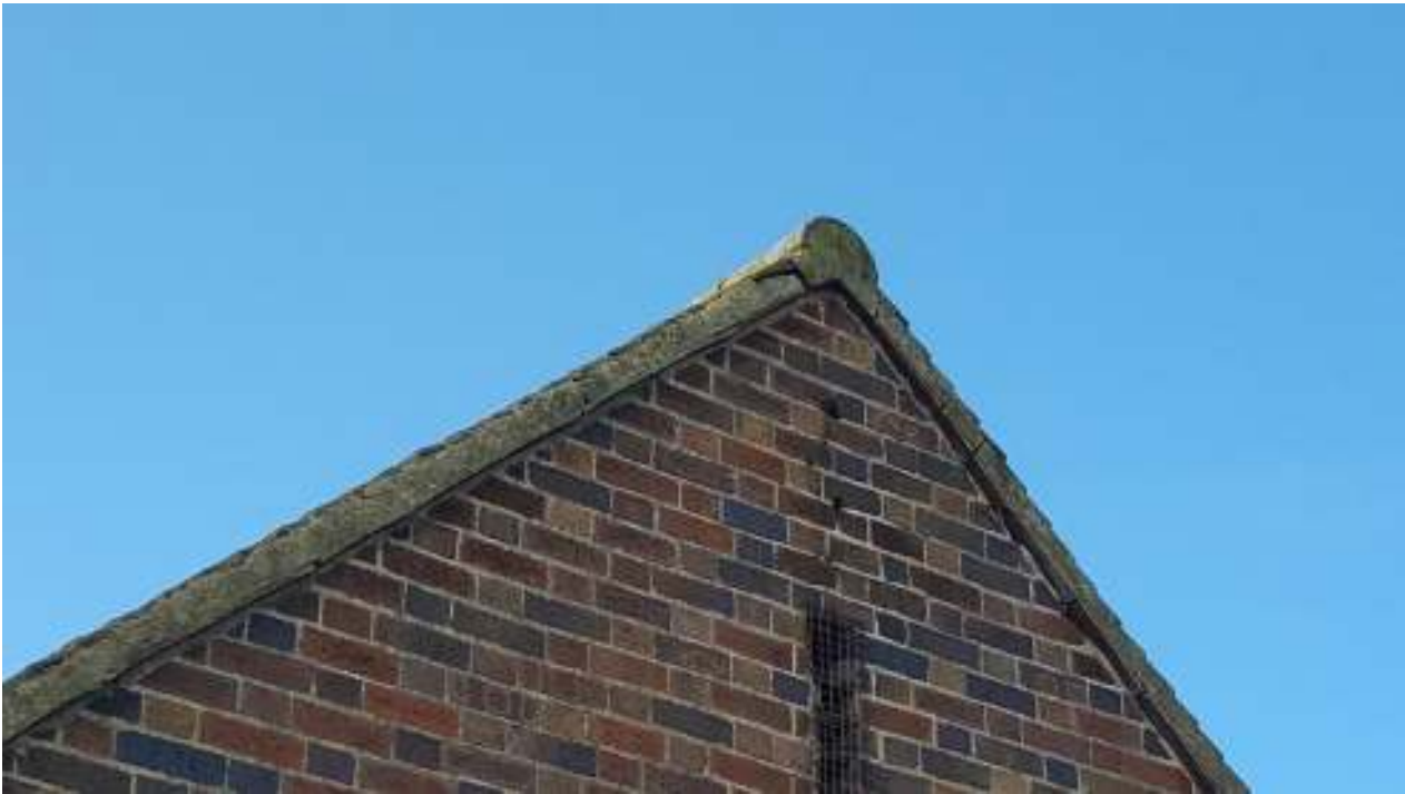
Plate 4: Showing B1 building crevice potential Bat access point
