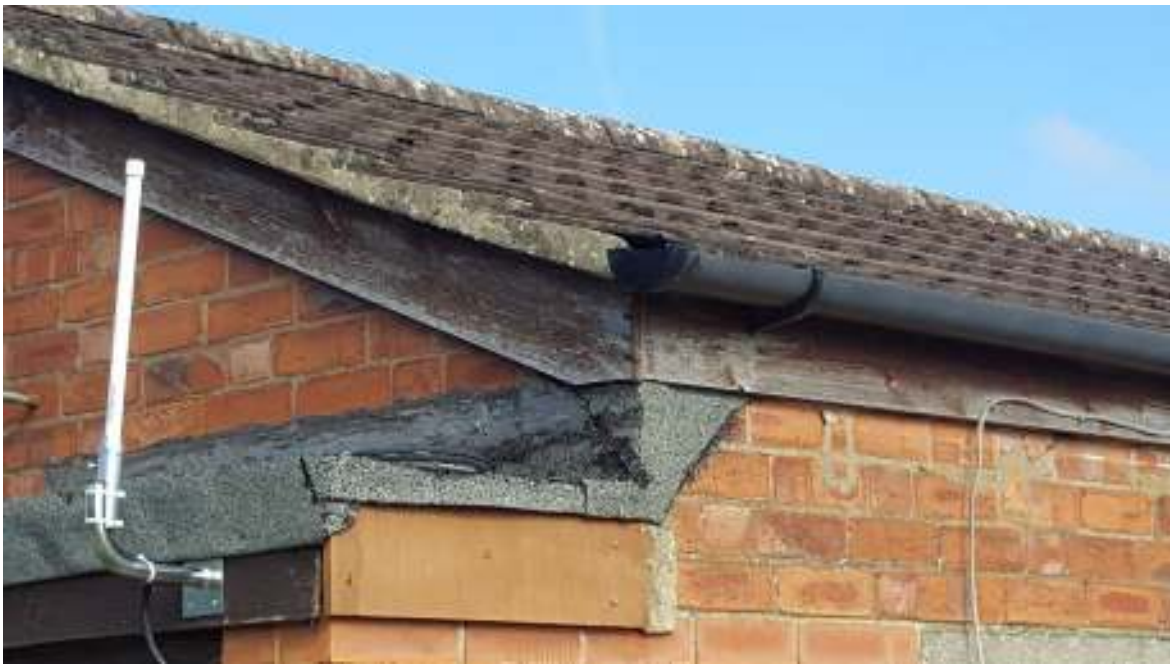
Plate 2: Showing B1 building crevice potential Bat access point.
