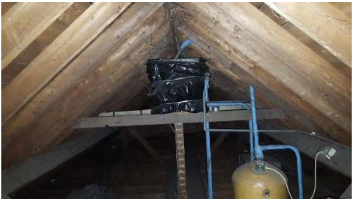
Plate 7: Showing roof void within B3
